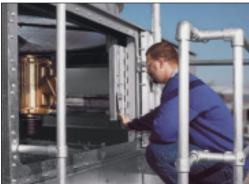
The T.E.A.O. fan motor is located inside the fan casing on the large AT Cooling Tower, and is mounted on a rugged heavy duty motor base. The motor base is designed to swing completely to the outside of the unit through a very large hinged (14 square feet) (1.3 square meters) access door greatly simplifying motor maintenance.
