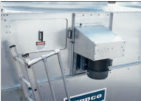
extended to the exterior casing and are located by the access door, thus making bearing lubrication easy.
